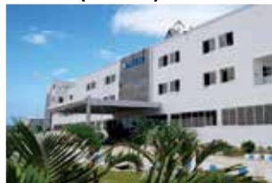
Rudrapur Plant (Green Building)
