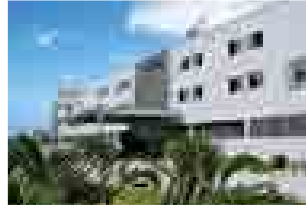
Rudrapur Plant (Green Building)
