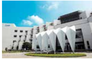
Tainan Plant (Diamond-rated Green Building)
