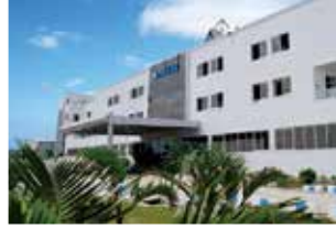
Rudrapur Plant (Green Building)
