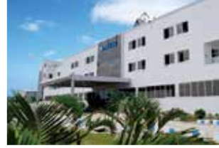
Rudrapur Plant (Green Building)
