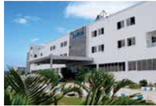
Rudrapur Plant (Green Building)
