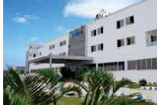
Rudrapur Plant (Green Building)
