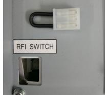
RFI Switch on the motor drive
