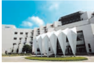
Tainan Plant (Diamond-rated Green Building)
