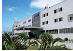
Rudrapur Plant (Green Building)
